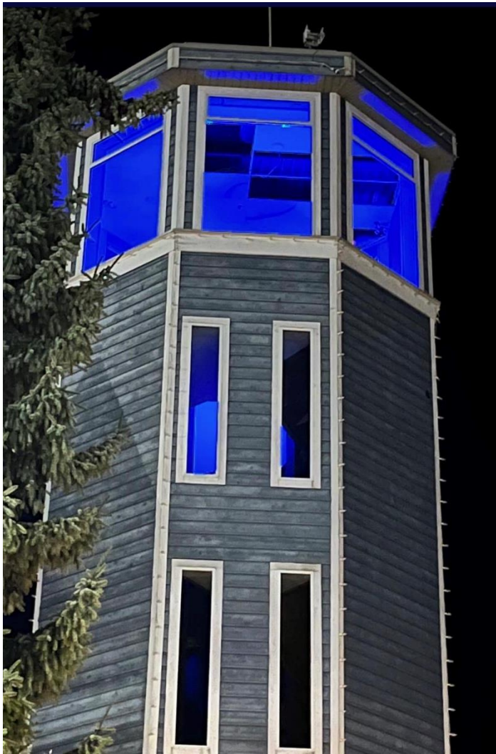
District of Sechelt Tower
