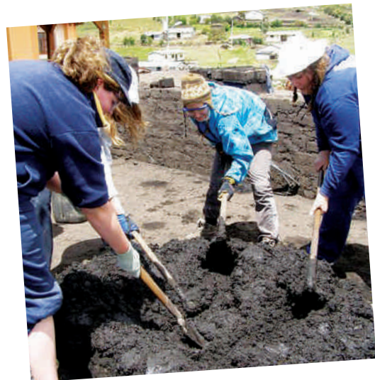
Building a school in Ecuador
